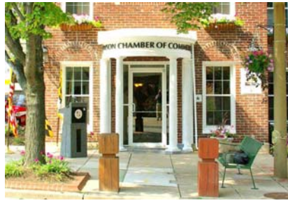
New Chamber Building
